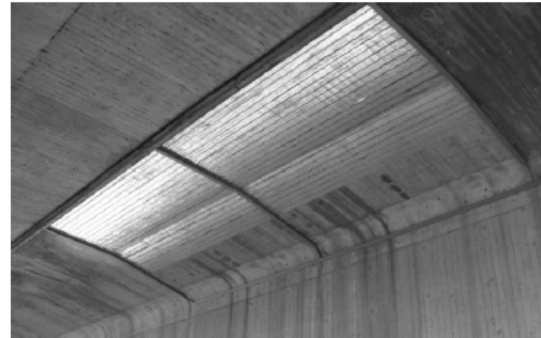
Figure 2. Zinc strips applied on section 2 and 3.
