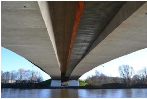
Figure 4. The access to the soffit at the damaged cantilever.
