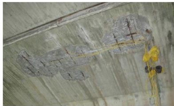
Figure 17. Repair locations and RE's in segment 3.
