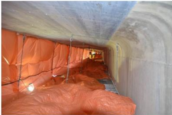
Figure 5. The workspace created underneath the bridge.
