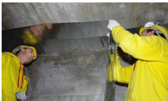
Figure 7. Application of the zinc anode in strips.
