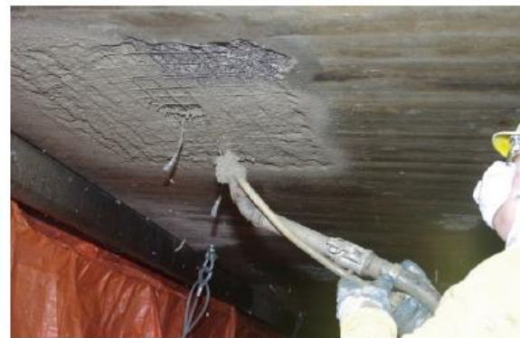
Figure 6. Repair of the damaged locations with shotcrete.
