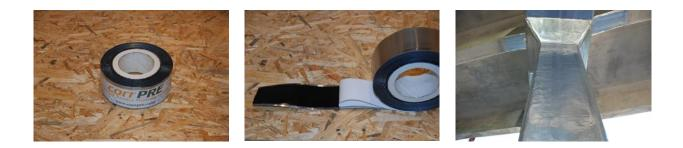
In case no waterproofing system will be applied it is recommended to seal all the exposed ends to avoid humidity ingress.
